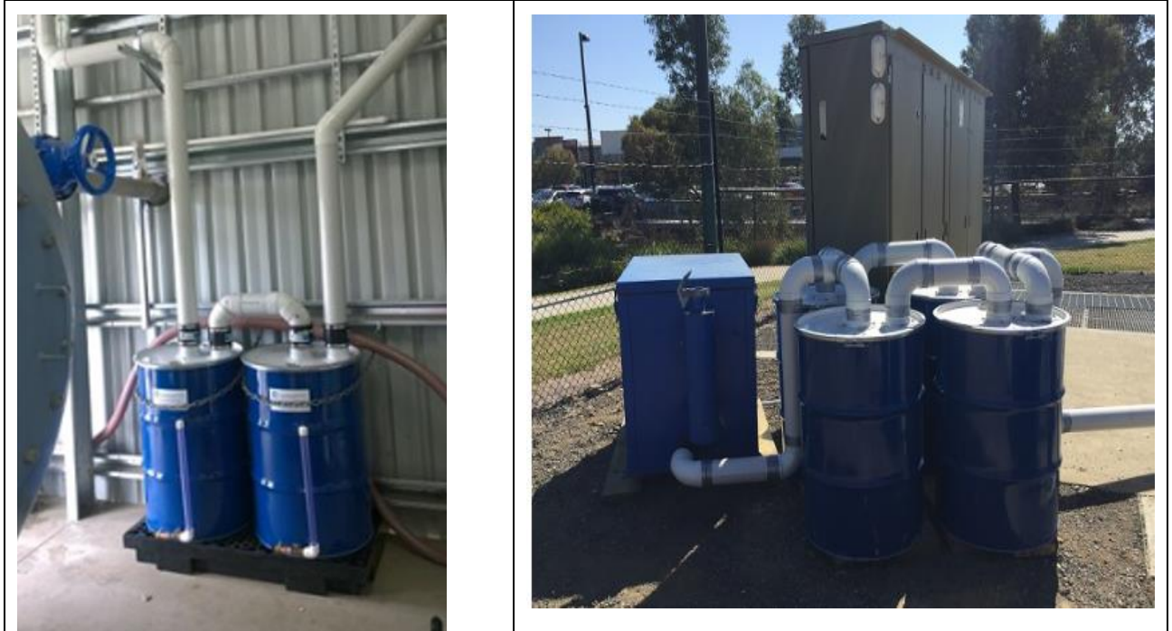
Figure 5.6: Granular Activated Carbon (GAC) Canisters for Air Filtration
